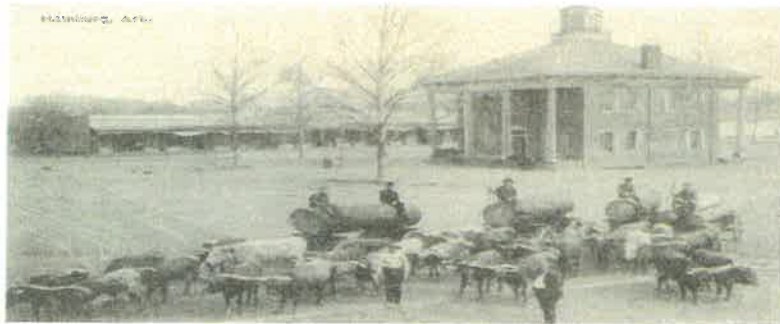
2 ND ASHLEY COUNTY COURTHOUSE – IT WAS DECIDED IT WAS NO LONGER ADEQUATE FOR USE IN 1903
